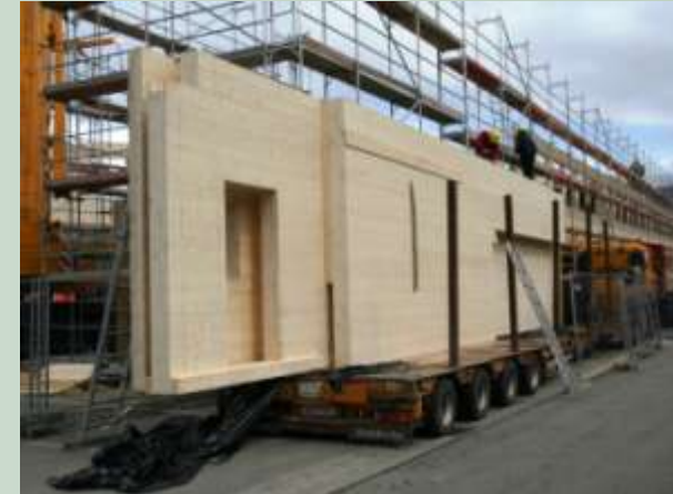
discharging (building site)
