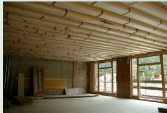
CLT/GLT ceiling element as a ripped base plate (span length 8 m)
