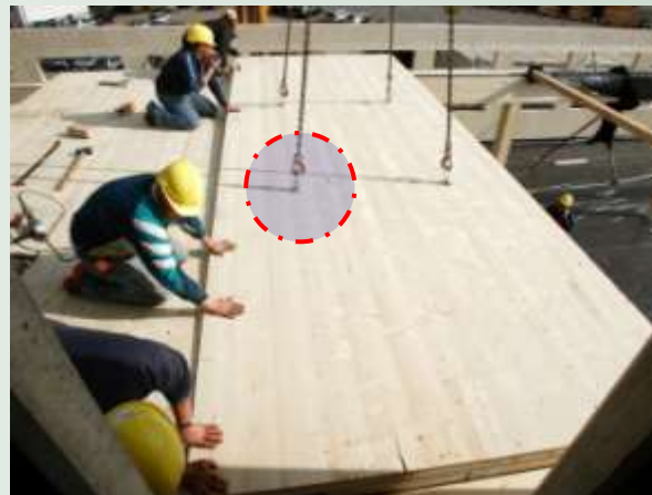
mounting parts for ceiling elements
