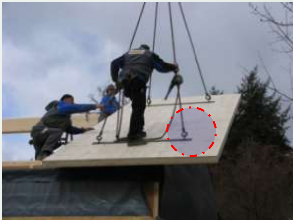
mounting parts for roof elements
