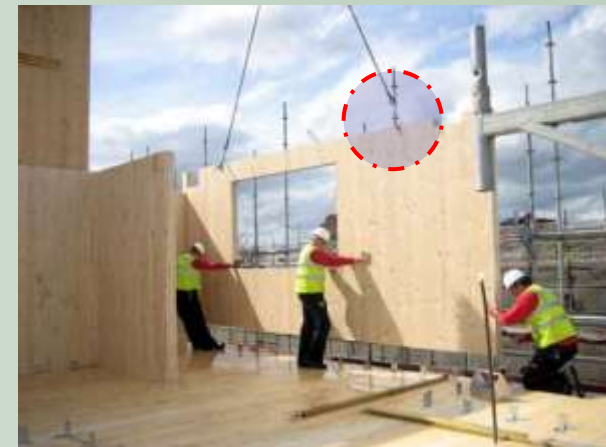
mounting parts for wall elements
