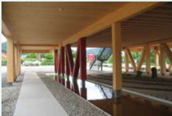
line supported CLT ceiling (with GLT beam)
