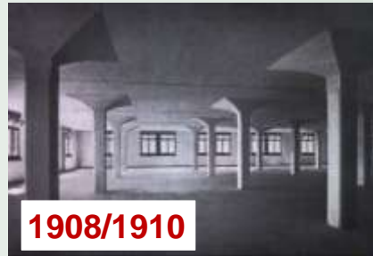
RC ceiling on enlarged column heads ("mushroom headed")
